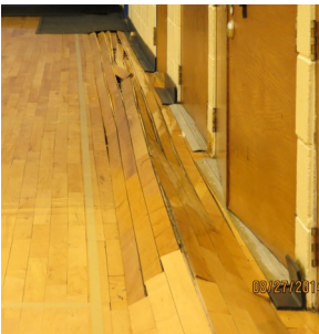
Construction in the summer, in a gym that did not have the HVAC system on and open doors allowed the humidity level to exceed typical acclimated humidity levels within the gym and expanded the wood floor—this was a temporary construction issue.
